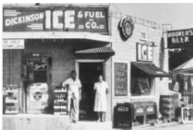
Dickinson Ice & Fuel Co. formed in 1922 and built the community's first water system.
